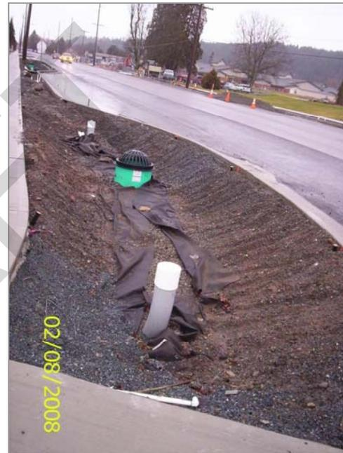
**Figure 4. Roadside Green Street /LID Application Under Construction**
