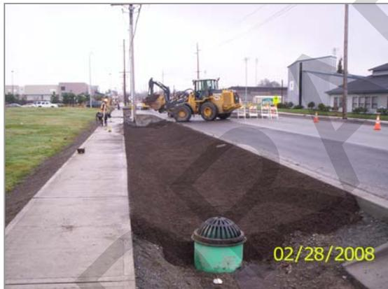
**Figure 3. Roadside Green Street /LID Application Under Construction**
