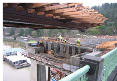
Bridge Construction on the New Sauvie Island Bridge
