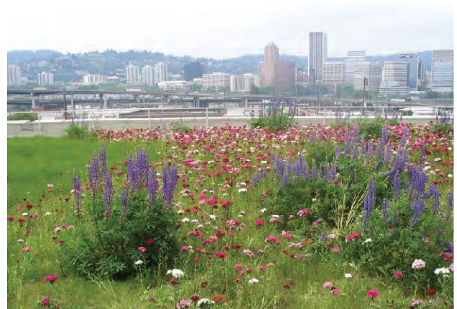
Multnomah Building Green Roof
