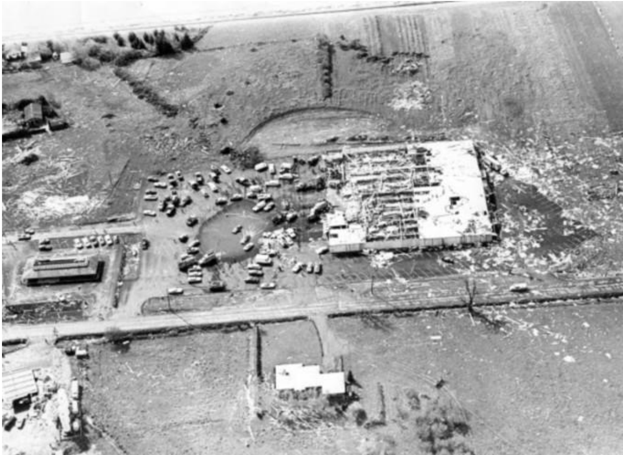
Figure 80 - Damage in Vancouver, Washington caused by the 1972 tornado. Photo and oral recount provided by Clark History.
